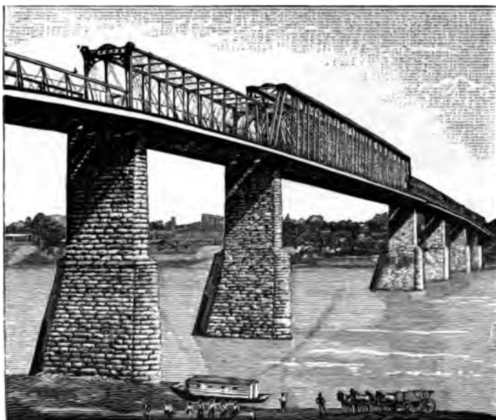
RAILROAD BRIDGE ACROSS THE OHIO RIVER.
